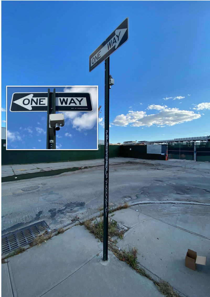
Figure 13: Street signpost mounted sensor in at 5th St and Hoyt St, in Gowanus. Inset shows front-facing closeup of sensor.
