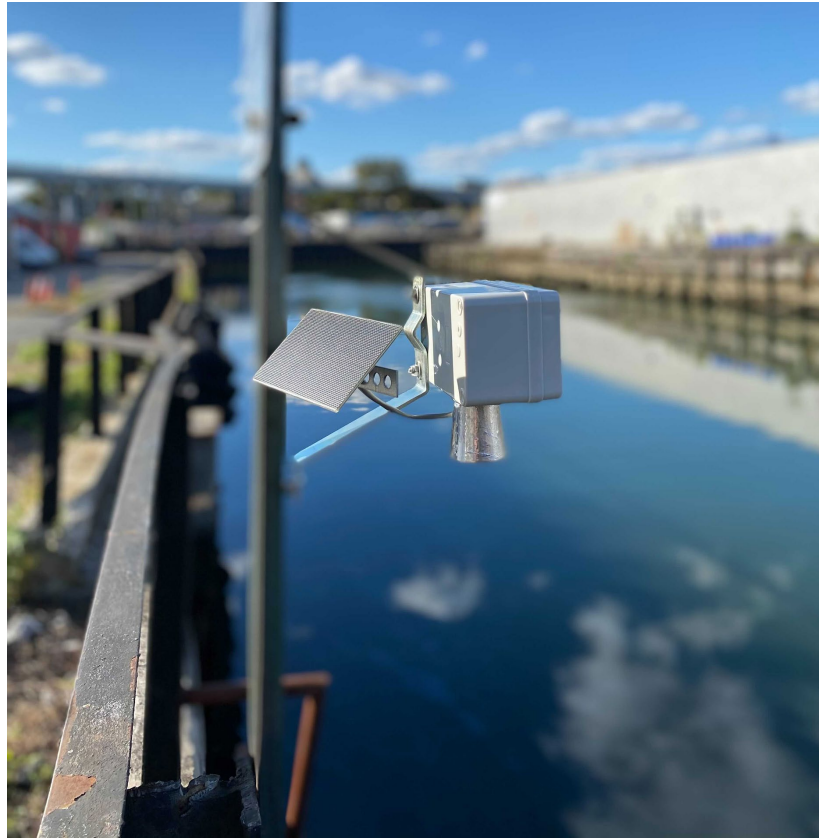
Figure 12: Gowanus Canal mounted distance sensor showing rear-mounted solar panel
