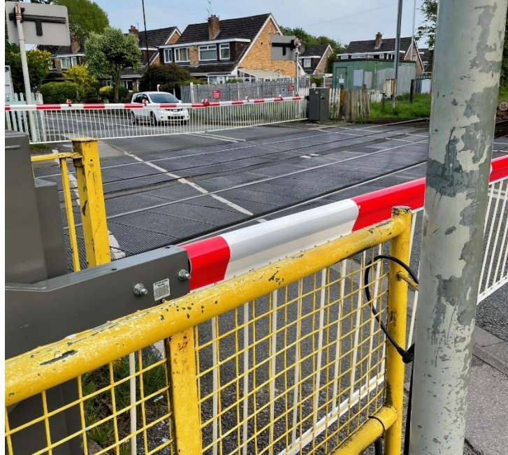
Figure 8: Metrolink crossing at Navigation Rd. Active warning extends over sidewalks and overlaps with fencing. Speed limit for Metrolink is 50mph (fieldnotes, 2023).
