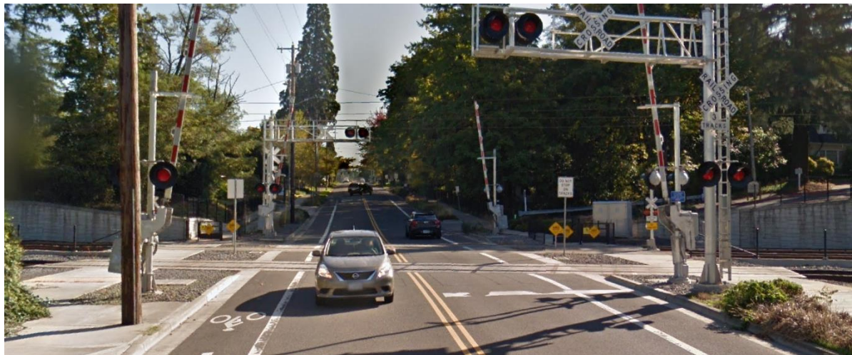
Figure 9: MAX at SE Harrison St. Grade crossing has quad gates, but no pedestrian control on near side (and only passive control, in the form of manually opened gates, on the far side). Speed limit for MAX is 30mph (Photo from Google Streetview).
