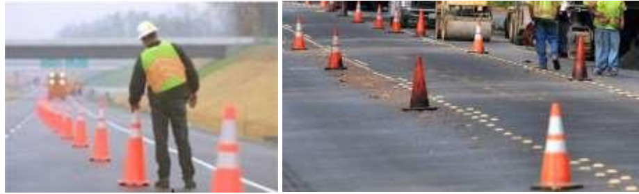
Figure 6 Example of a worker setting up cones.
