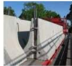
e) Portable Concrete Safety Shape Barrier (PCBs)
