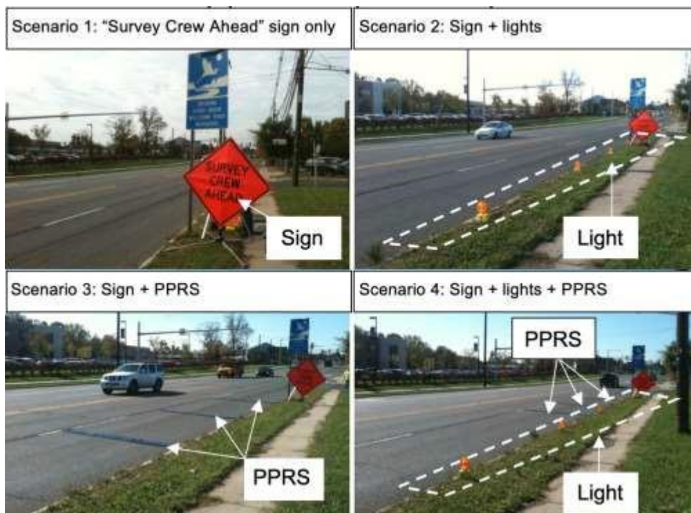
Figure 13 Different Traffic Control Devices used for surveyors' work (mobile work zone)
