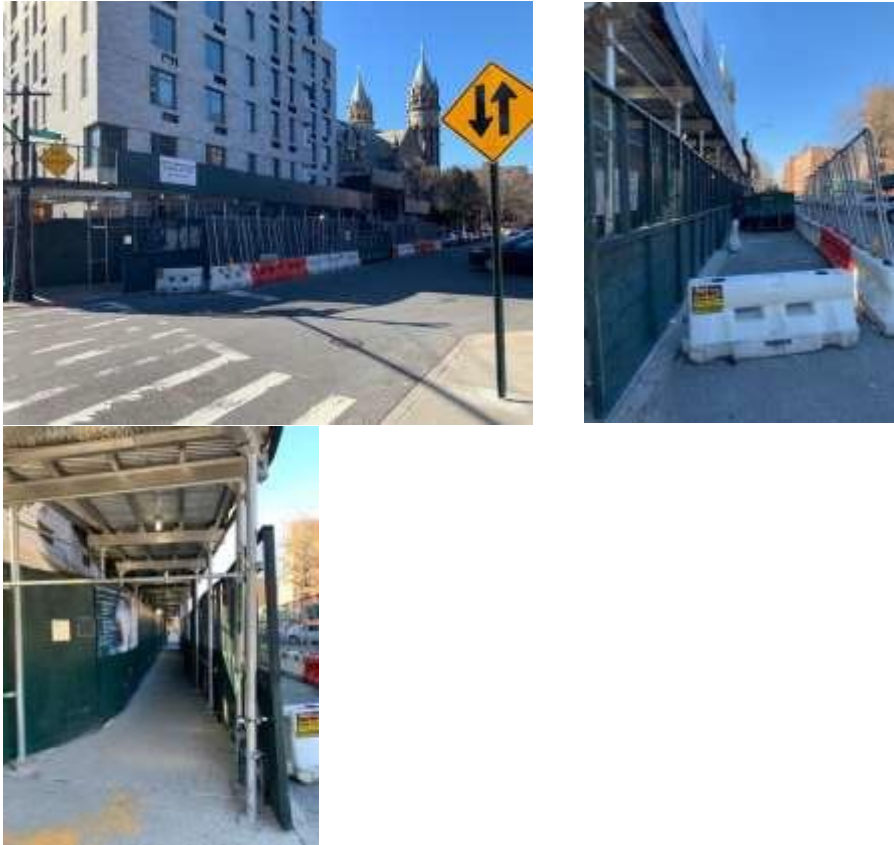
Figure 17 Work zone condition captured using a camera for scenario one.
