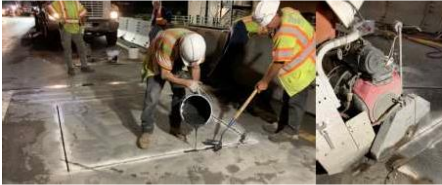
Figure 8 Example of workers finishing installing a weight sensor.
